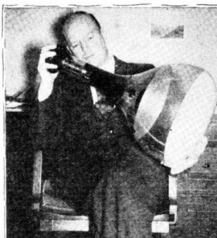
Newest (American) Dumont 12-inch cathode-ray receiving tube - 1937-'38.
