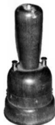
MEUCCI'S TELEPHONE-IM. M=Magnet. D=Diaphragm. C=Coil and ear plate.
